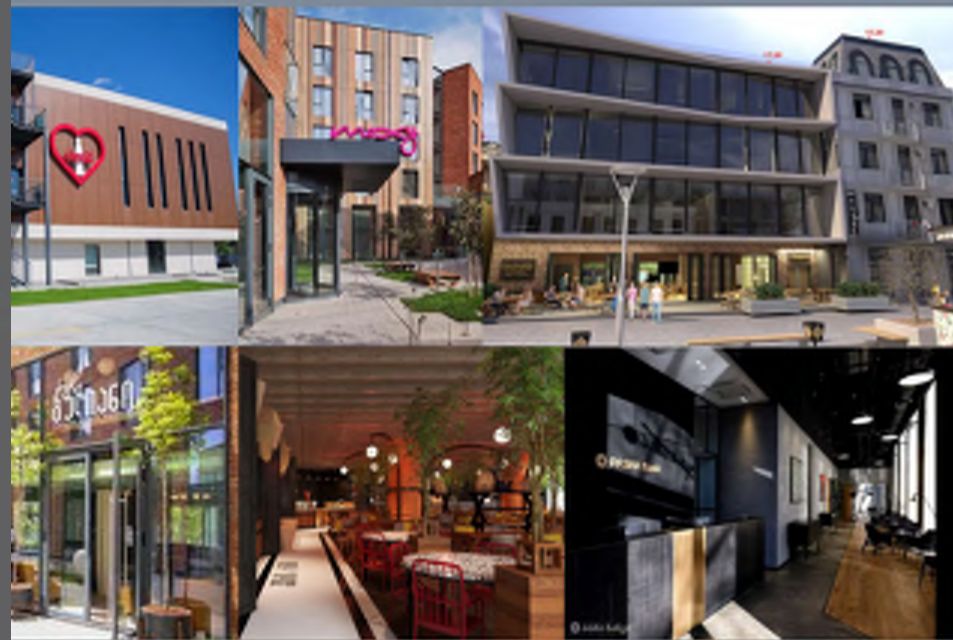
JSC. "Medical Corporation Evex" office complex (MEP)
